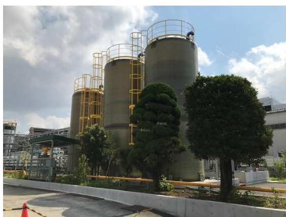
*1 Appearance of newly installed facility
